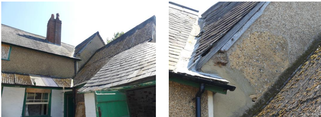
Figs. 12 & 13 Roof tiles and verge
