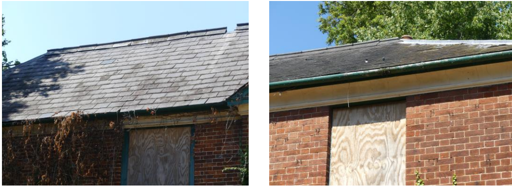
Figs. 10 & 11 Ridge and roof tiles
