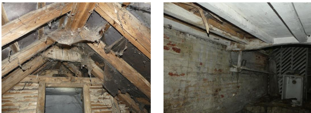
Figs. 18 & 19 Roof void (L) and cellar (R)
