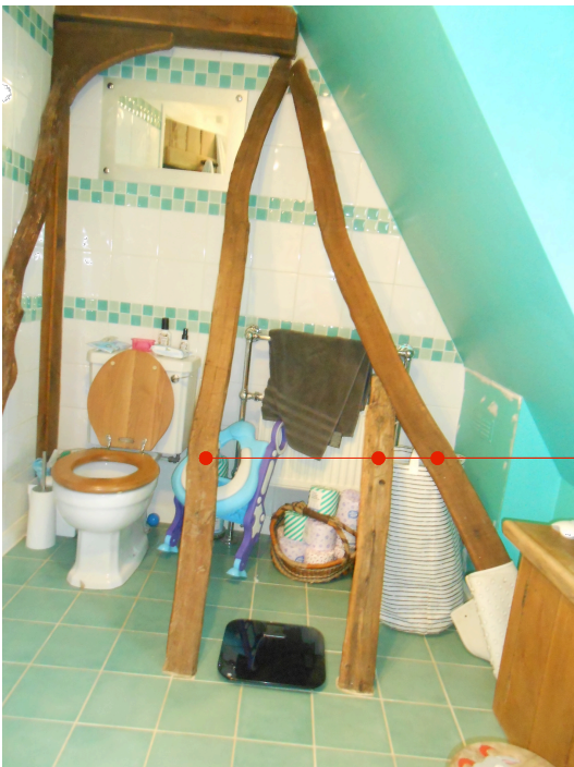
Photograph 1 - First Floor bathroom
