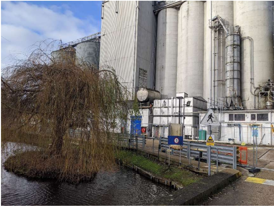
5. Derelict mill buildings.
