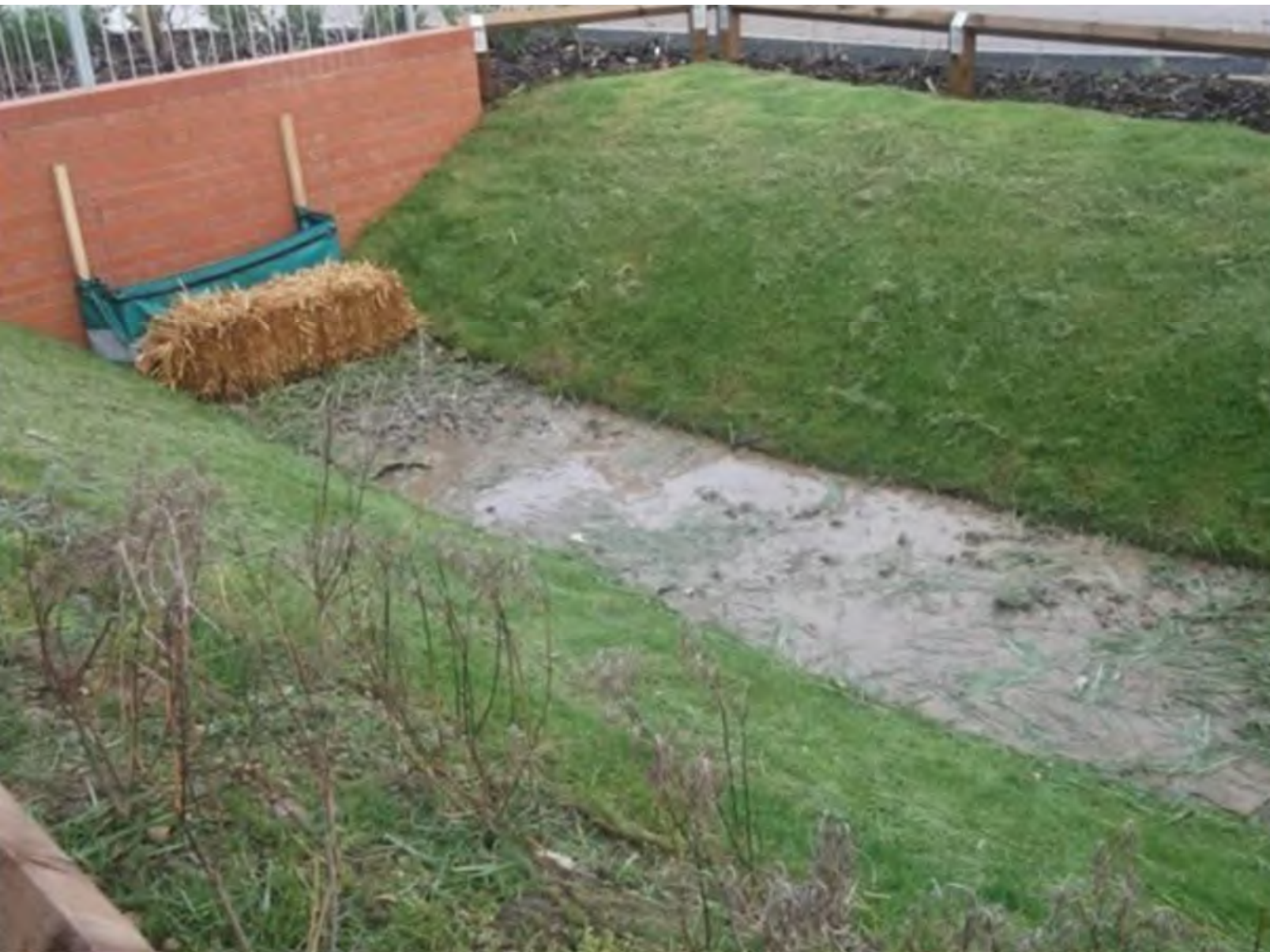
Example of installation of silt fencing with straw bales at a headwall within a swale
