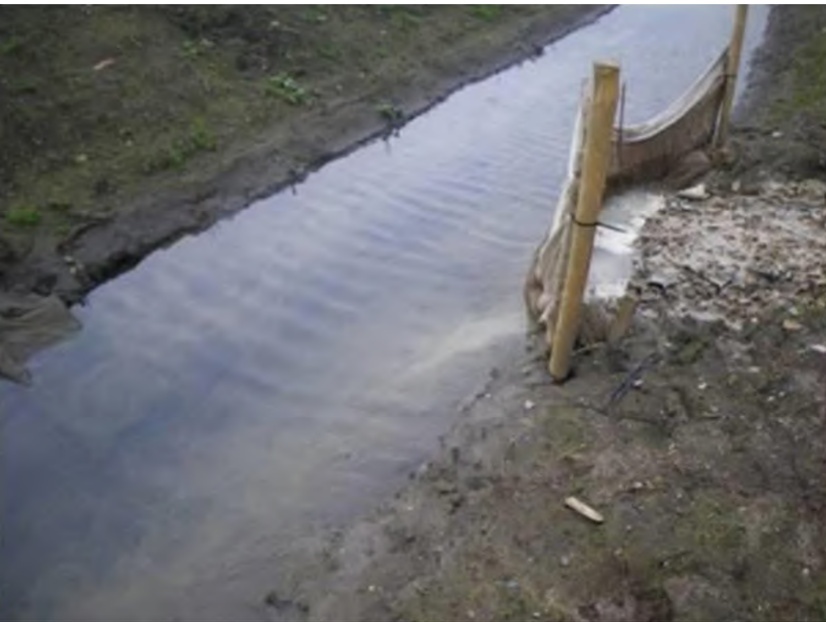
Example of silt matting to intercept run-off
