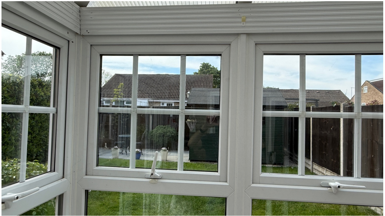
Figure 5: View of Existing Roof (at 23 Kipling Close) from our Conservatory
