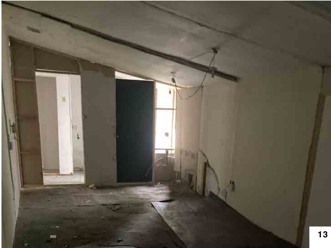
Existing in-fill building interior
