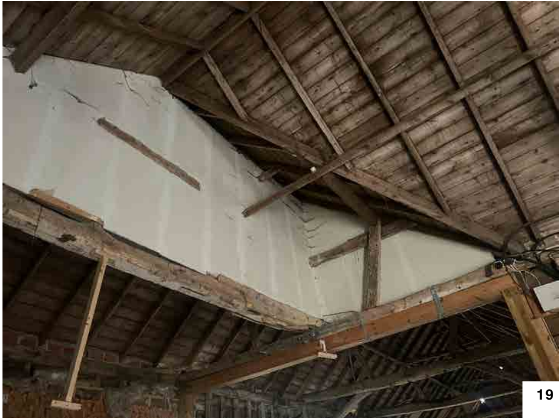
Historic barn - outside of the scope of the project
