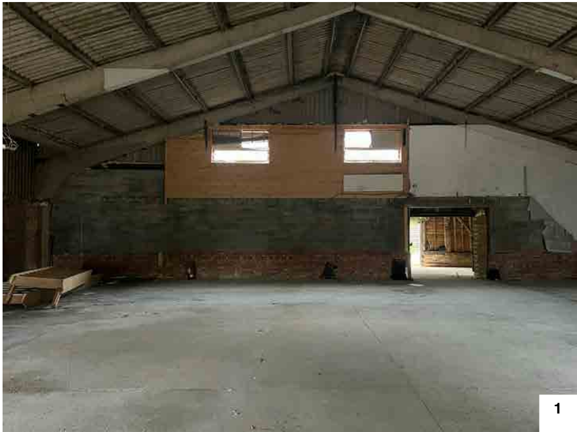
Concrete barn - interior
