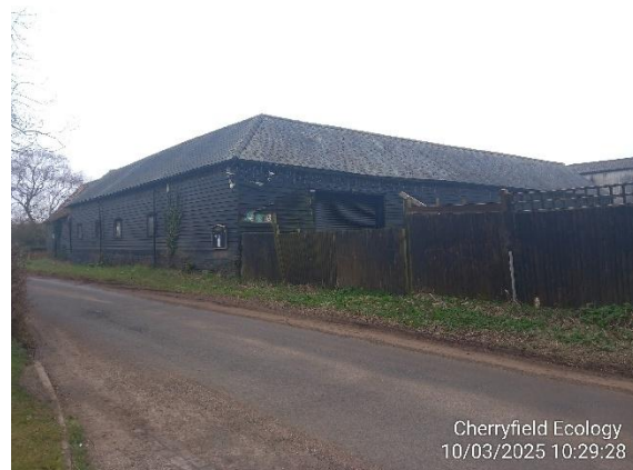
Figure 5: Example of B2's northeast exterior
