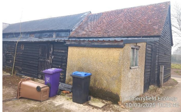
Figure 7: Example of B2's southwest exterior
