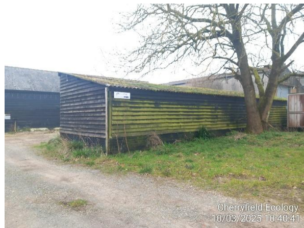
Figure 13: Example of B5's exterior
