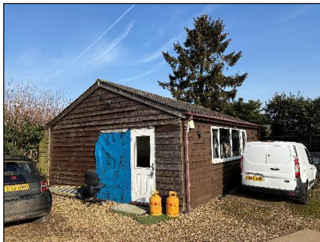
Photograph 5 Southern and eastern elevation of outbuilding to north-west of site
