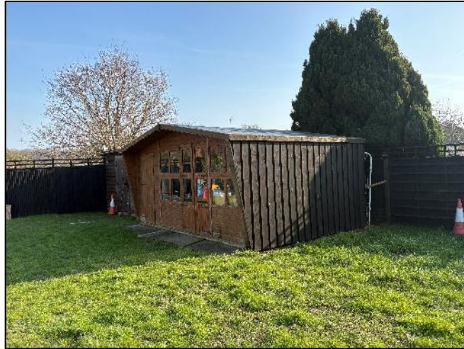
Photograph 4 Southern and western elevations of outbuildings to north-east of site
