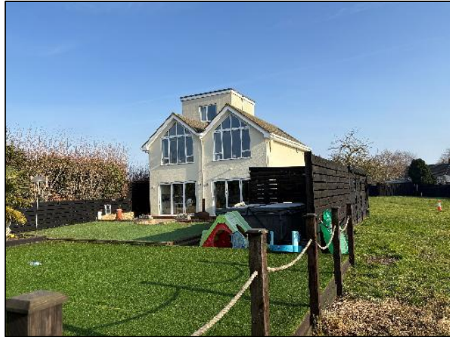
Photograph 1 Southern elevation of residential property and artificial grass to the south
