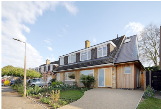
front view of 87 Westwood Avenue
