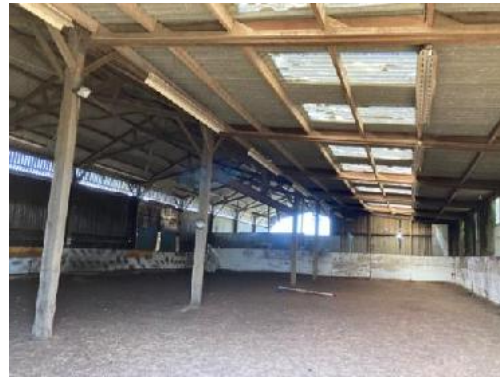
Photograph 14: Internal of Building B2
