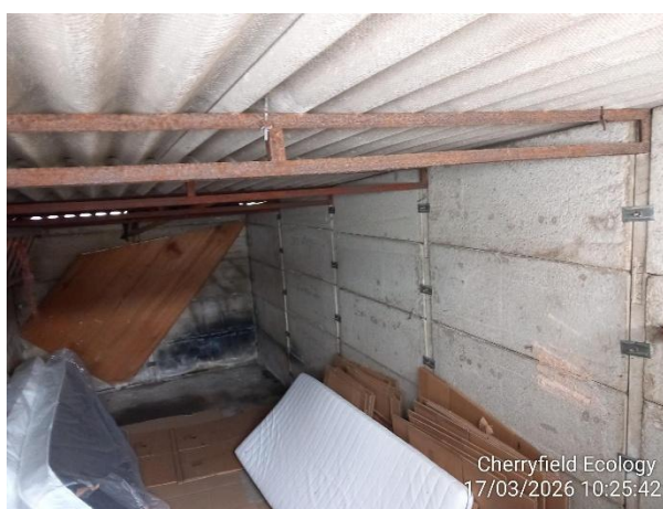
Figure 8: Another example of B2's interior
