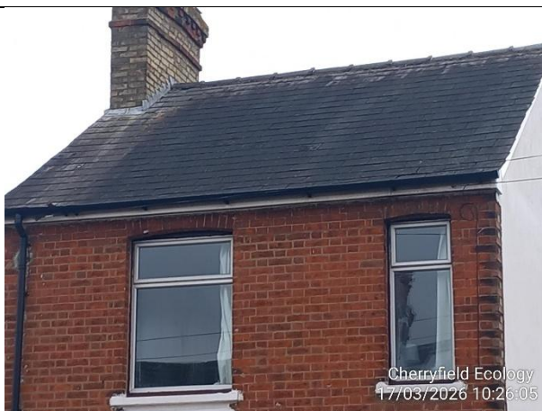
Figure 9: Example of the tightly fit slate roofing tiles
