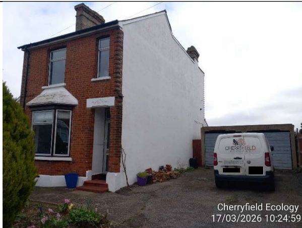
Figure 2: Example of B1's front exterior
