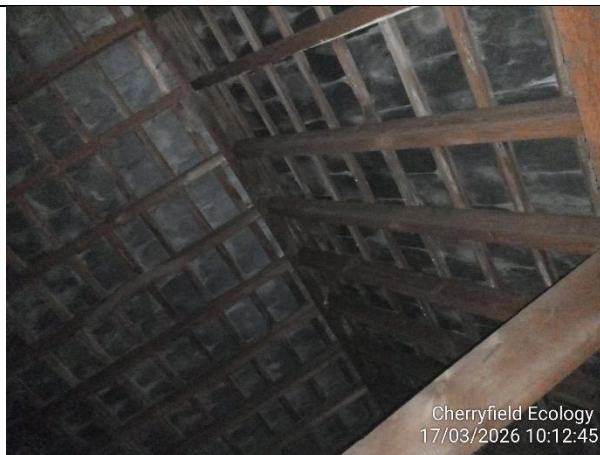
Figure 5: Another example of B1's interior
