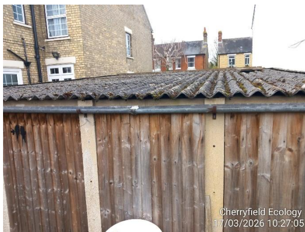
Figure 6: Example of B2's exterior
