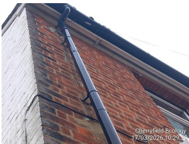
Figure 10: Example of the tightly fit soffit box
