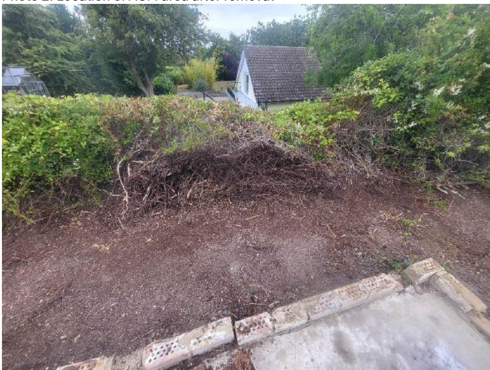
Photo 2: Location of ACM area after removal
