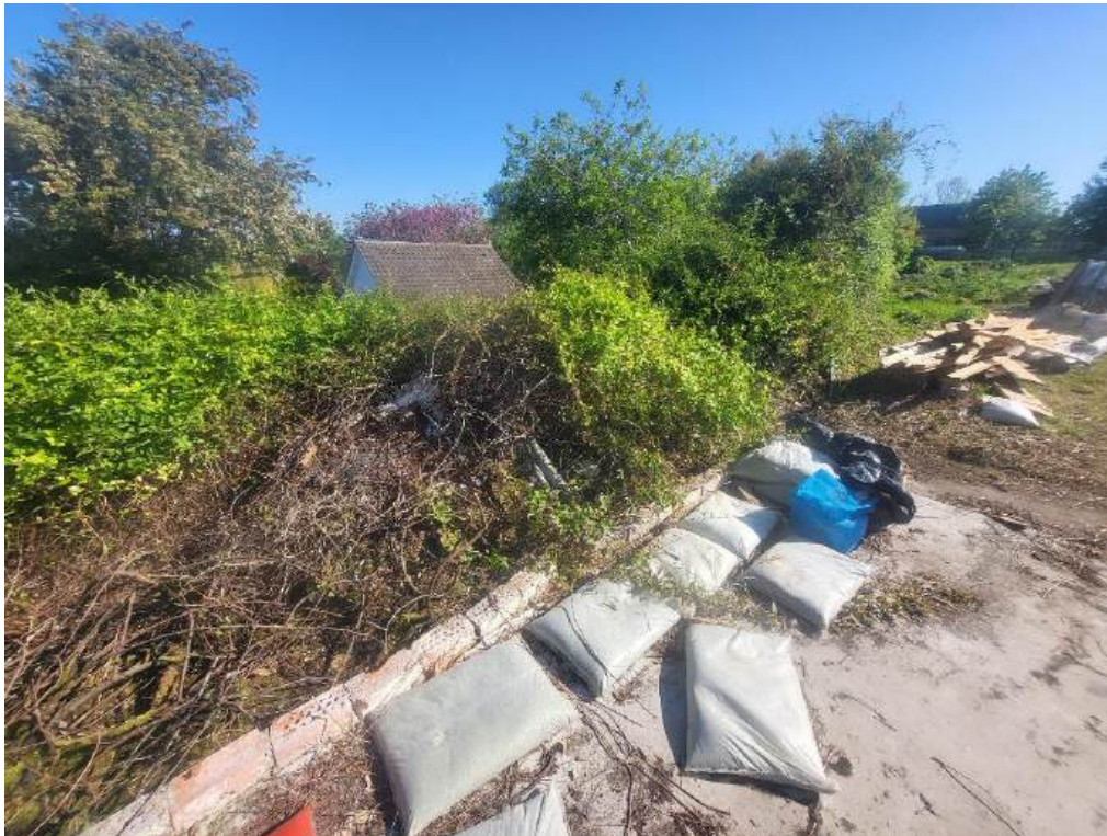
Photo 1: Location of ACM pile before removal
