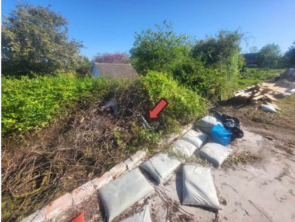
Photo 3 - Stockpiled asbestos cement sheeting
