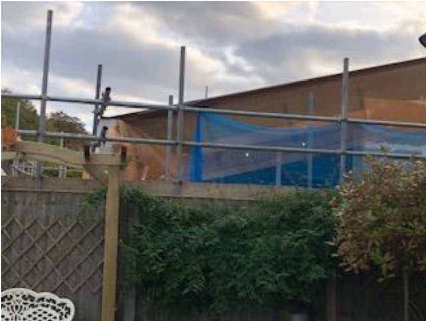
Image 6. View from back garden of 24 The Warren showing upper part of living room window of 15 Garden Lane. Again, scaffolding and netting obscures full view.
