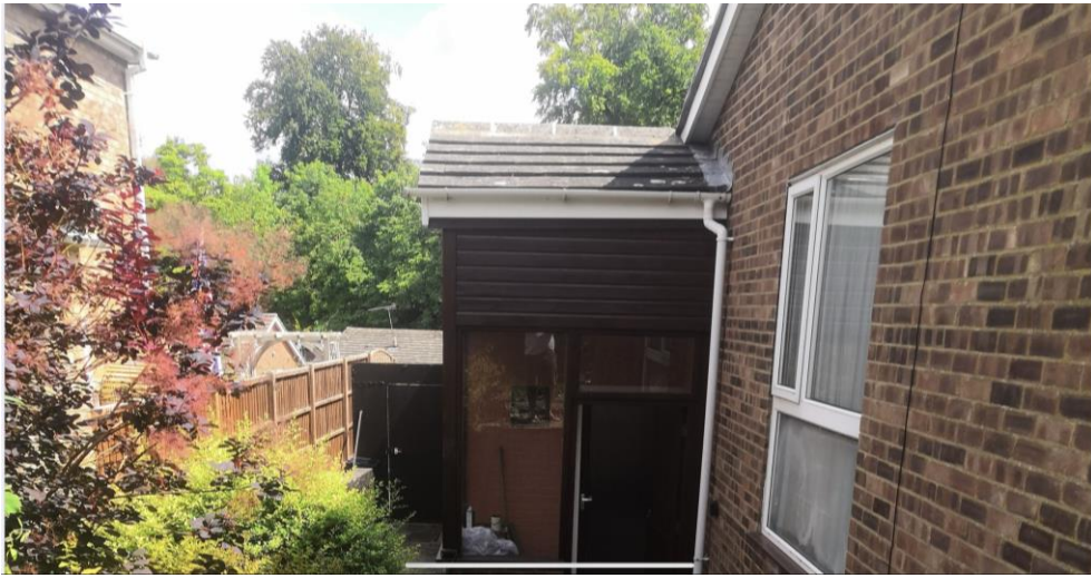
Image 7. Original non-obscure window of 15 Garden Lane facing 24 The Warren garage wall and angled view to kitchen.
