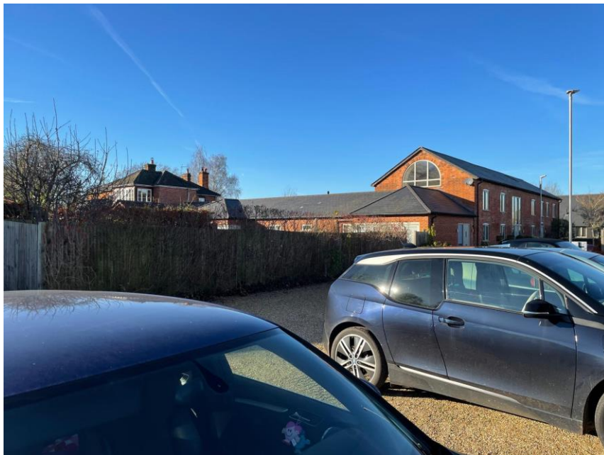
D – View from the proposed parking to the north west demonstrating a brick facade with high level gable window.
