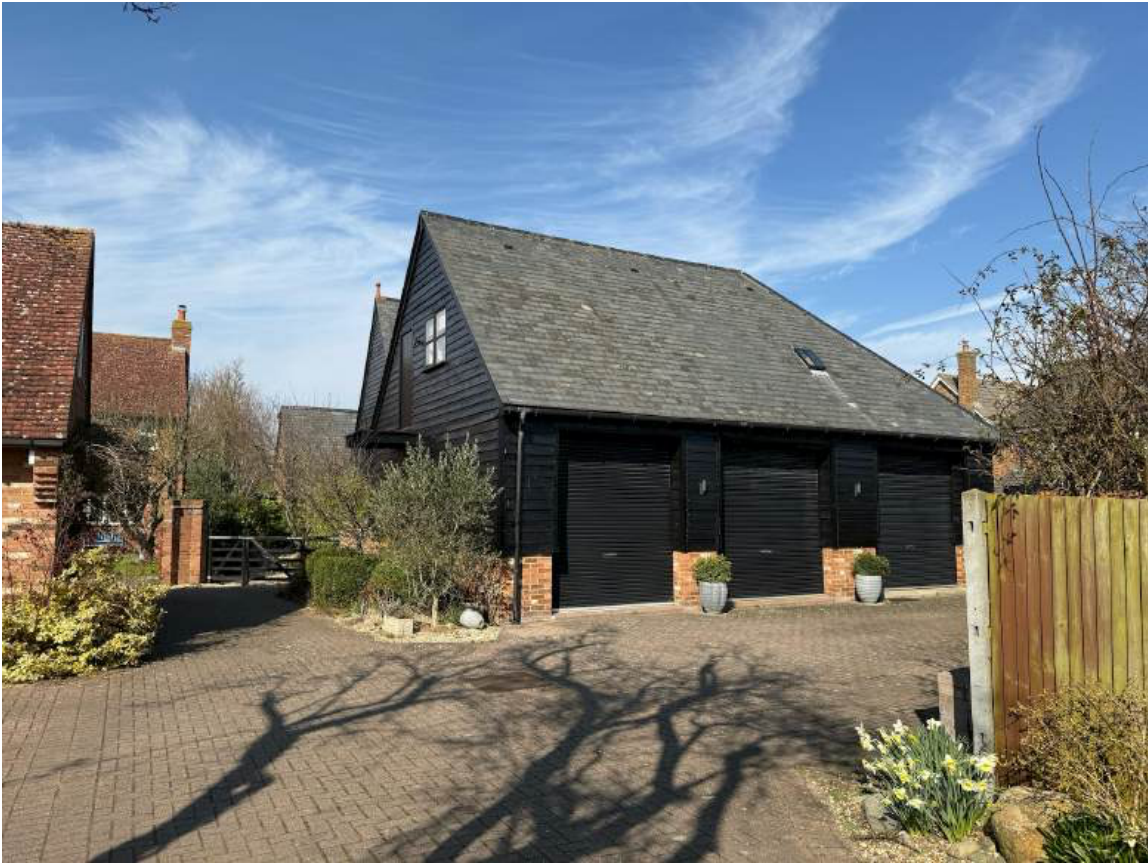
Number 33 behind. Garage to be clad in black timber to match
