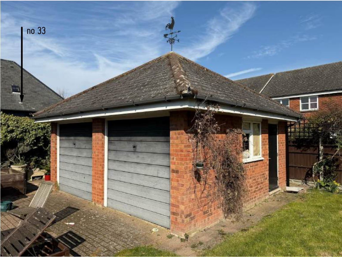
Garage to be converted to home office
