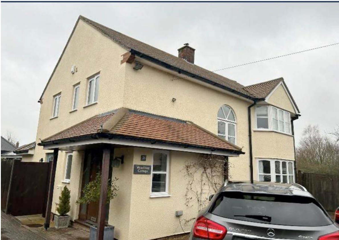
Existing yellow render and white windows to be repainted in heritage colours
