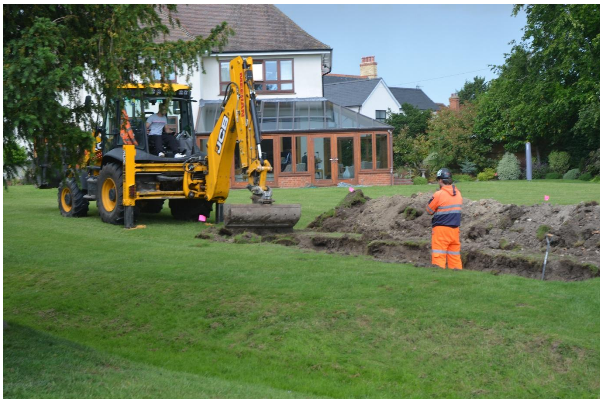
Plate 10. Machine excavation of Trench 3. View: Northwest.
