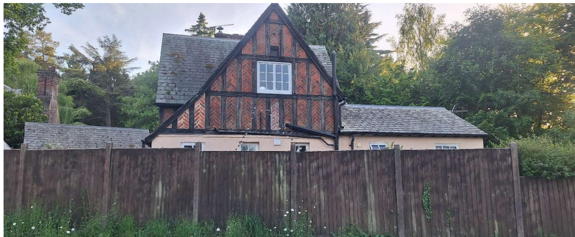
Photograph 11: View from opposite side of Preston Road. Potential survey location.
