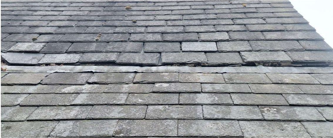
Photograph 9: Example of lifted slate tiles, sufficient to provide roost space for bats. Eastern aspect, Building A.
