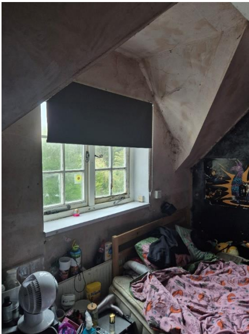
Picture 6 and 7 – Unventilated roof void, and lowered eaves sections and demonstration of existing mould and the external arrangements of dormers that creates cold bridging.
