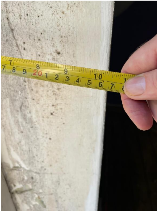
Picture 2 – Wall thickness demonstrated.
