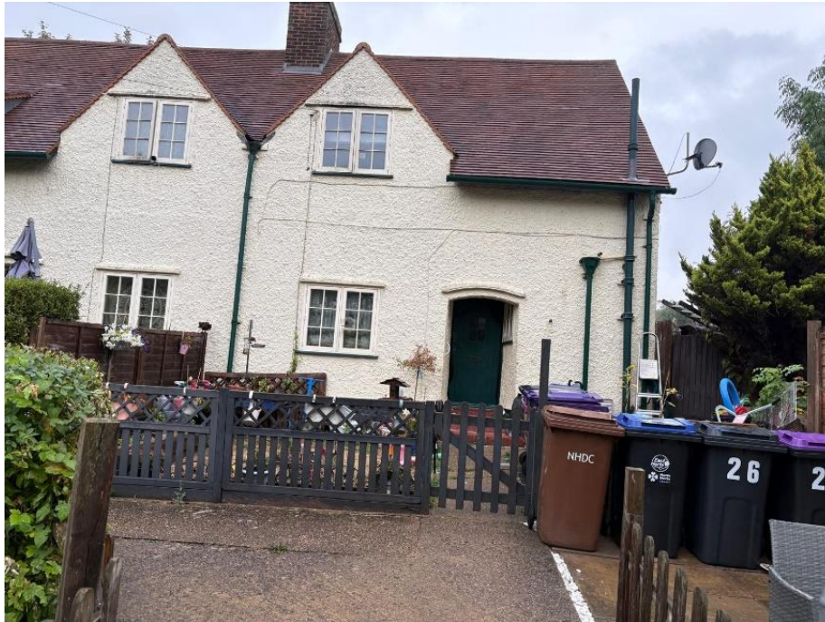
Picture 1 - Row of terraces representing the application, number 24 is the structure to the right of the central drainpipe..
