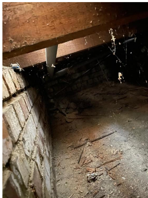
Picture 3 and 4 – Ventilation and clearly ventilated void of neighbouring buildings, buildings built in same period, matching footprints and assumed similar.
