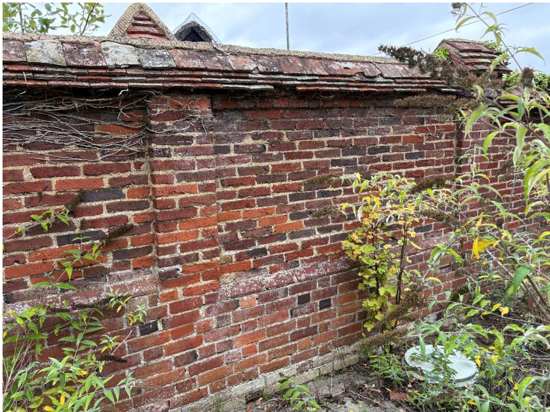
Wall viewed from Mill side
