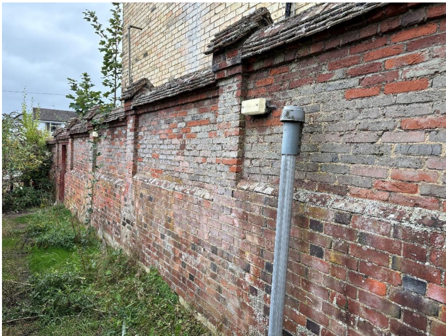
Boundary wall viewed from East Lodge side, Mill building behind
