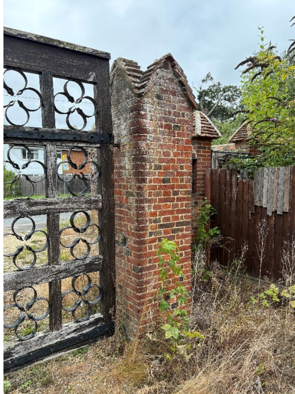
Entrance gate pier with gable coping detail
