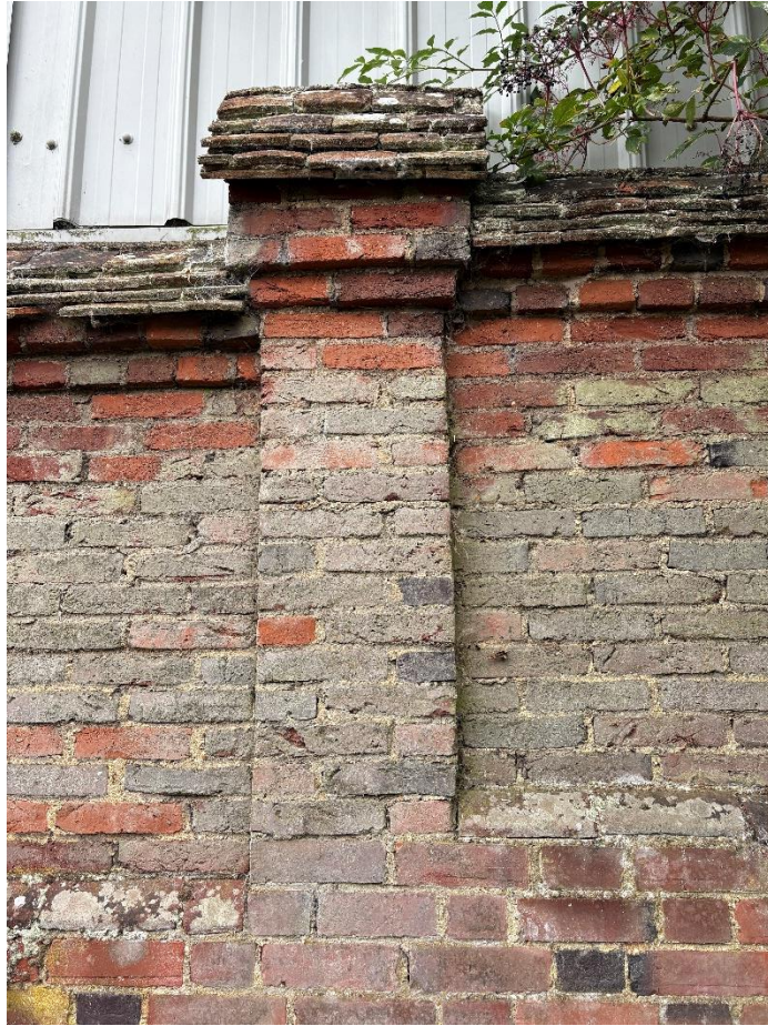
Pier and coping detail to boundary wall
