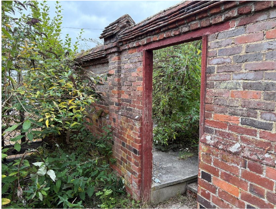
Pedestrian gate through boundary wall
