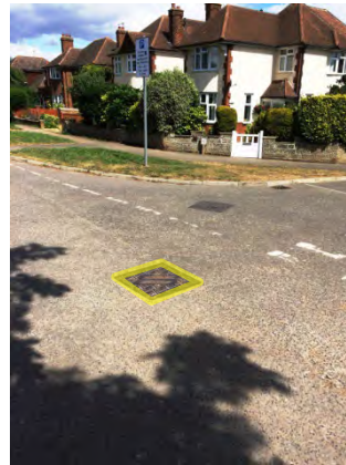
Manhole, on Lucas Lane, used as survey datum
