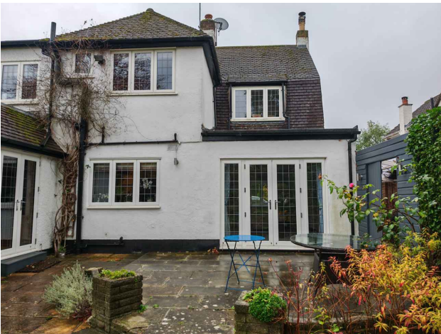
Rear Area to be Infilled for new Ground and first Floor Extensions
