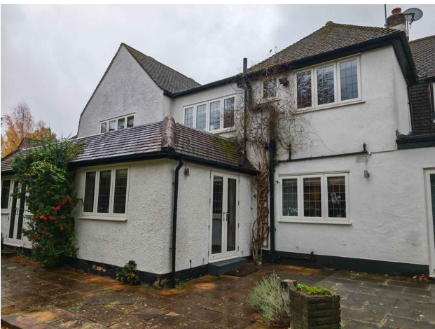
Existing Rear Elevation and Existing Rear Extension
