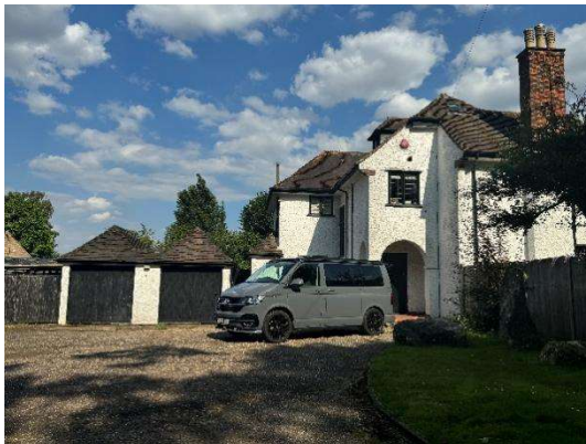
The existing house
