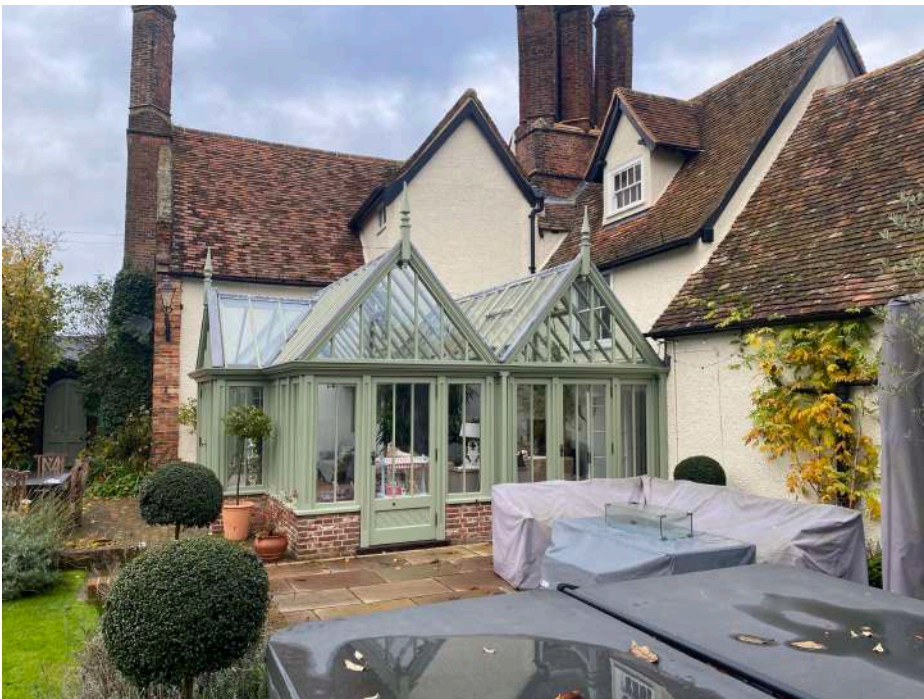
Photograph of the rear showing the existing haphazard arrangement of modern and old tiles
