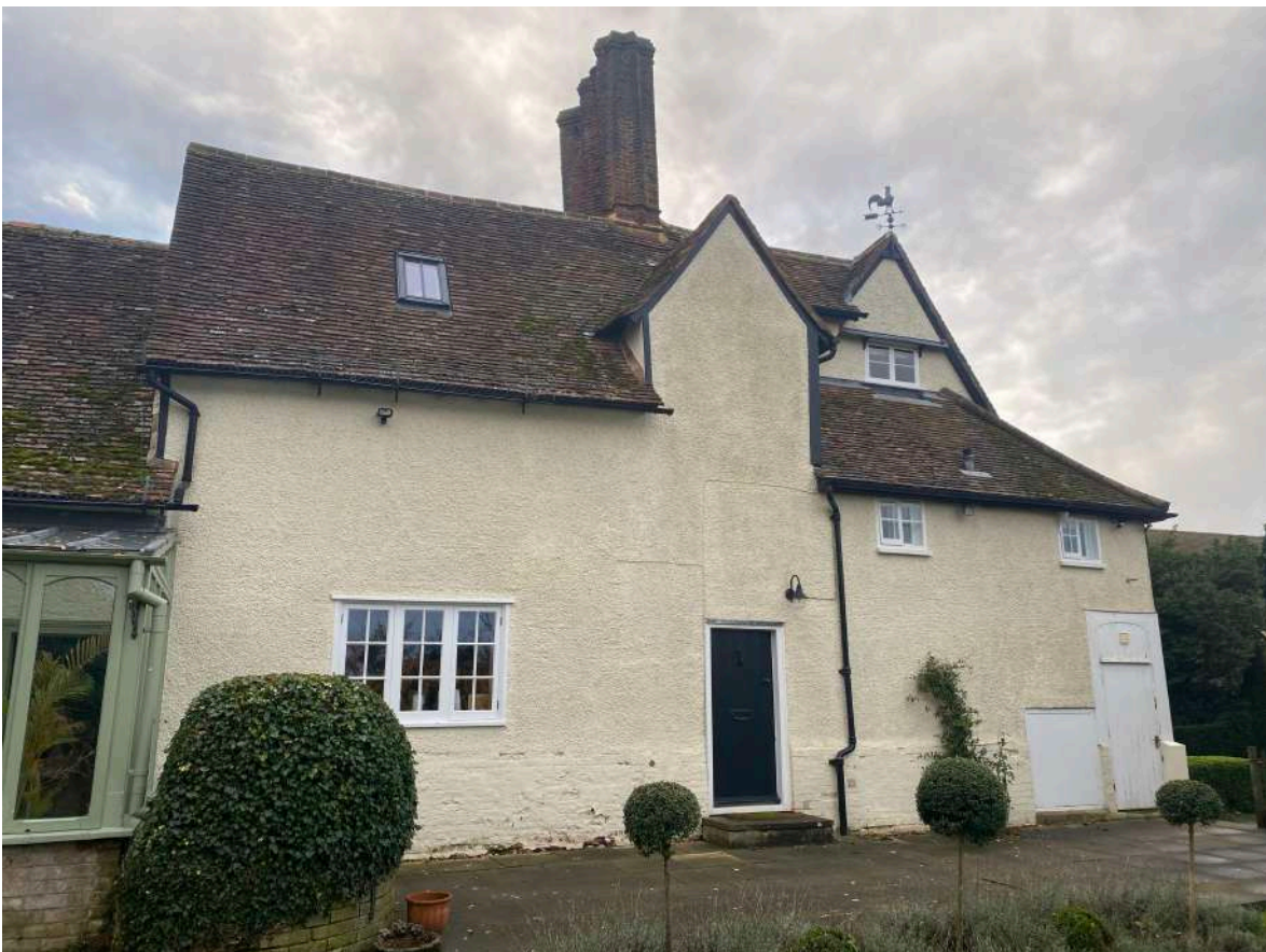
Photograph of the stair tower where the proposed roof light is to be installed
