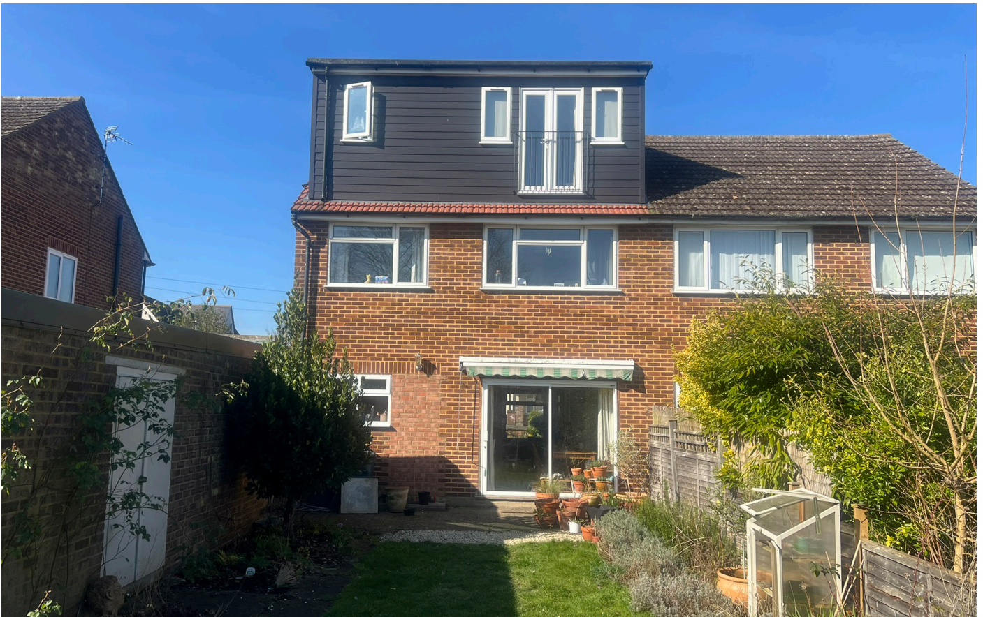
2. Existing rear view
