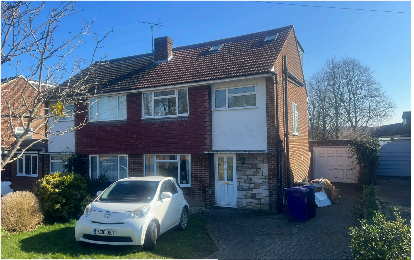
1. Existing front view
