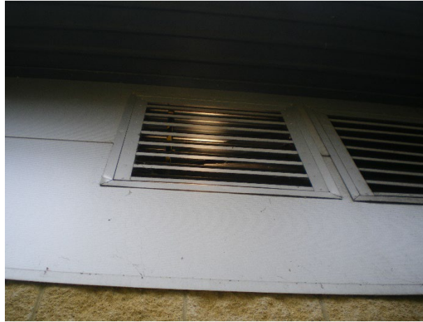
Feature 10: Vents on the wall. East elevation
