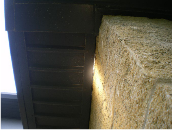
Feature 5: Small cavity between roof and overhang. North elevation on west side of the building
