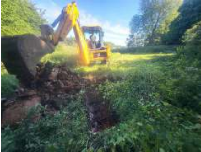
Photo 1: TP1 being excavated with JCB
