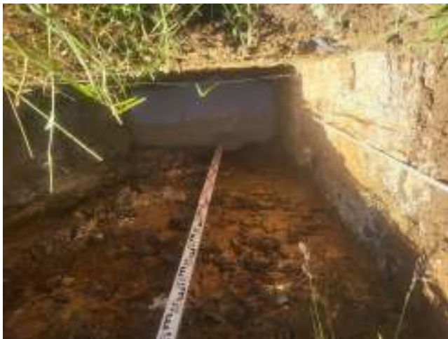
Photo 3: TP2 filled with water
