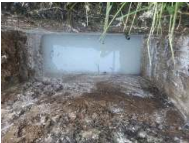
Photo 2: TP1 filled with water
