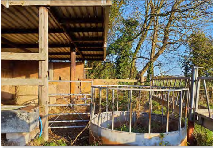
Building 1 Interior view from southern elevation. Photograph taken 04/12/2024.
