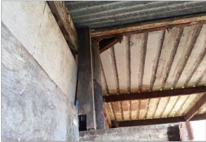
Building 1 Interior view of roof and western elevation wall. Photograph taken 04/12/2024.
