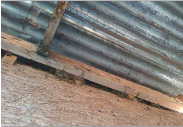
Building 1 Interior view of roof and southern elevation wall. Photograph taken 04/12/2024.
