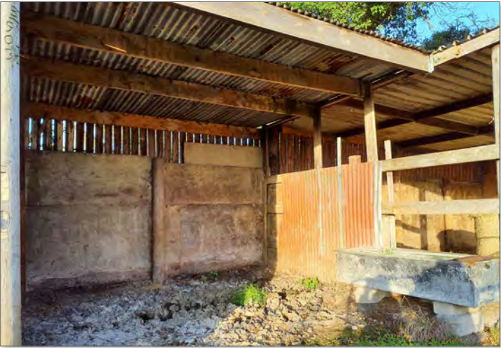
Building 1 Interior view from eastern elevation. Photograph taken 04/12/2024.
