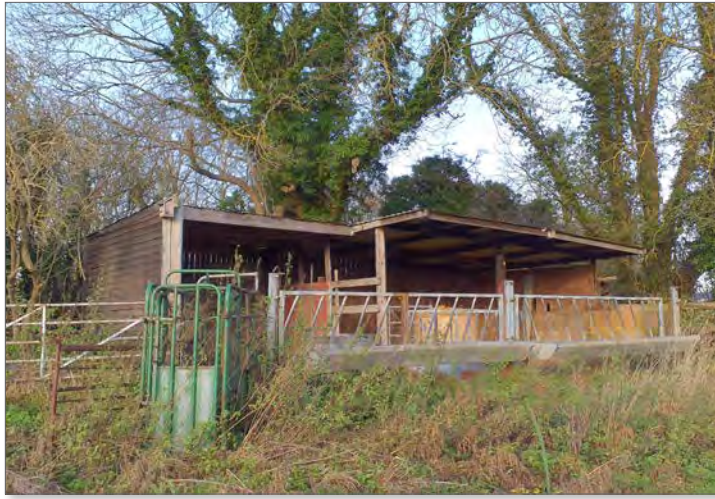
Building 1 Eastern elevation Photograph taken 04/12/2024.
