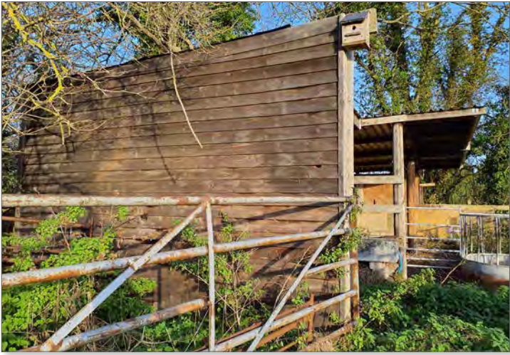
Building 1 Southern elevation with bird box shown. Photograph taken 04/12/2024.
