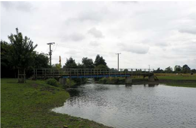
Arlesey Common Footbridge
