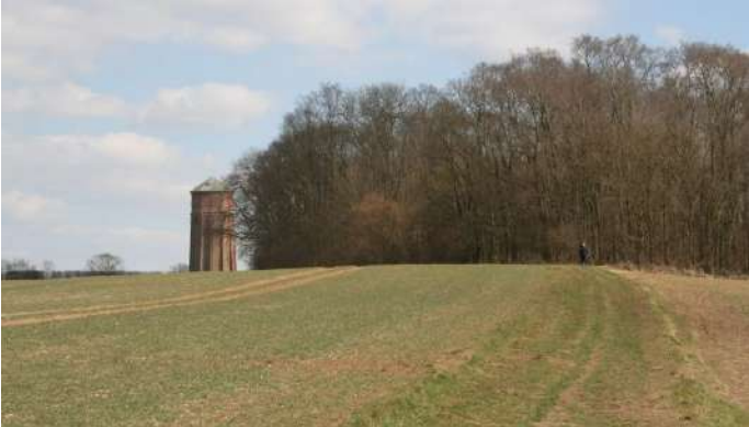
Linton Water Tower - an architectural feature against the woodland
