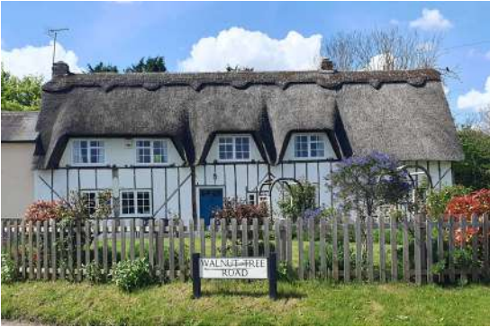
4-6 Walnut Tree Road - Grade II Exposed timber frame with plastered panels and distinctive thatch roof.
