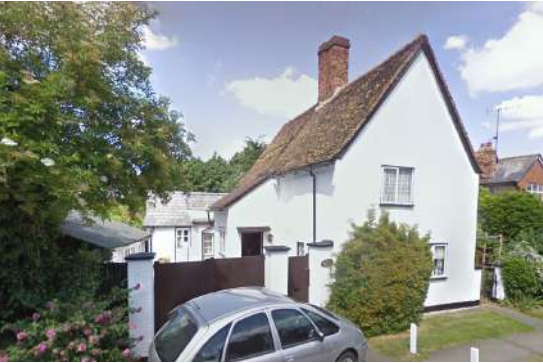
Arnolds Farm - Grade II Timber frame roughcast with black stuccoed plinth and steep tiled roof. Gable end presents a stark, monolithic facade to roadside.
