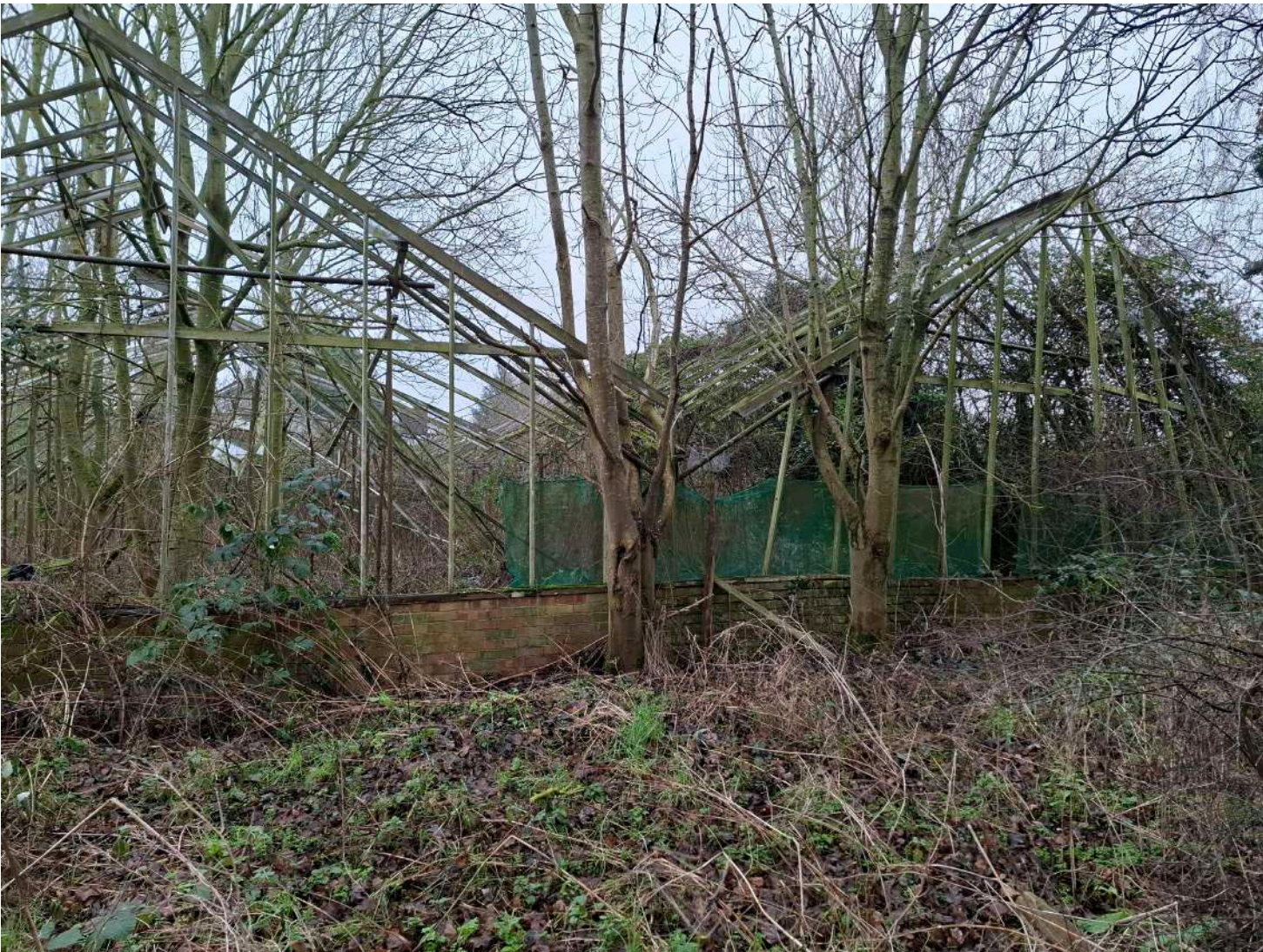
Disused nursery structures
