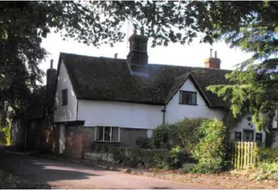
Tudor Cottage - Grade II Roughcast timber frame with ground floor cased in red brick. Jettying gables to first floor and irregular roof forms to southern elevation.
