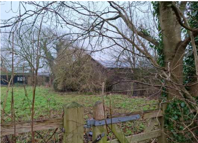
A600 Bedford road showing overgrown hedgerows and litter in verges (top) and dilapidated barn structure with ivy (bottom)
