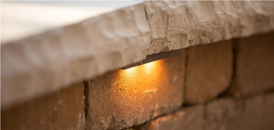
Figure 6 - Surface mounted outdoor LED lights to provide low level illumination on garden pathways and courtyard areas.
