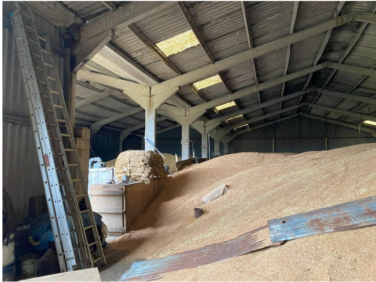
Photograph 3: Interior view of existing agricultural buildings (grain and machinery stores) for proposed change of use.
