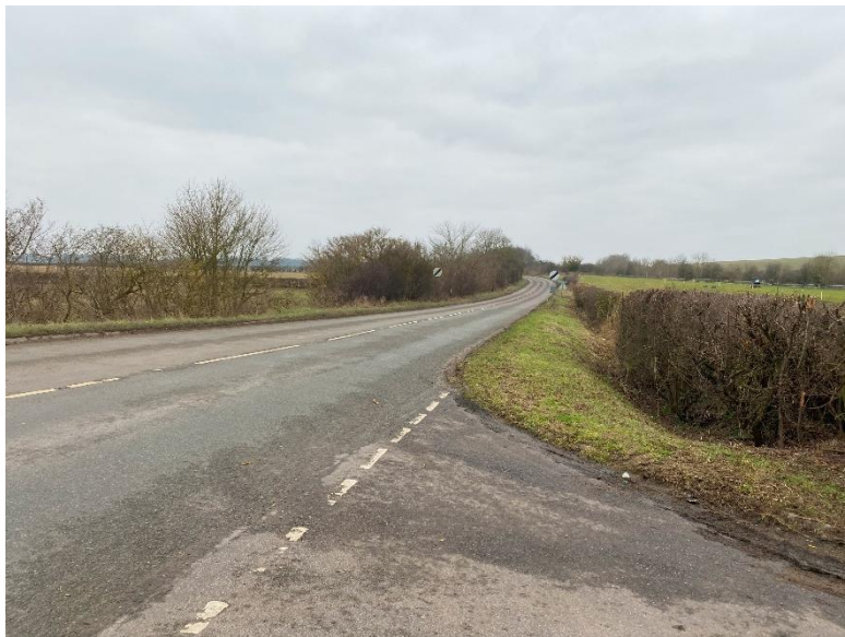
Photograph 8: Drivers eye view looking southwest from Lilley Hoo Lane junction with Hollybush Hill/Luton Road showing visibility.
