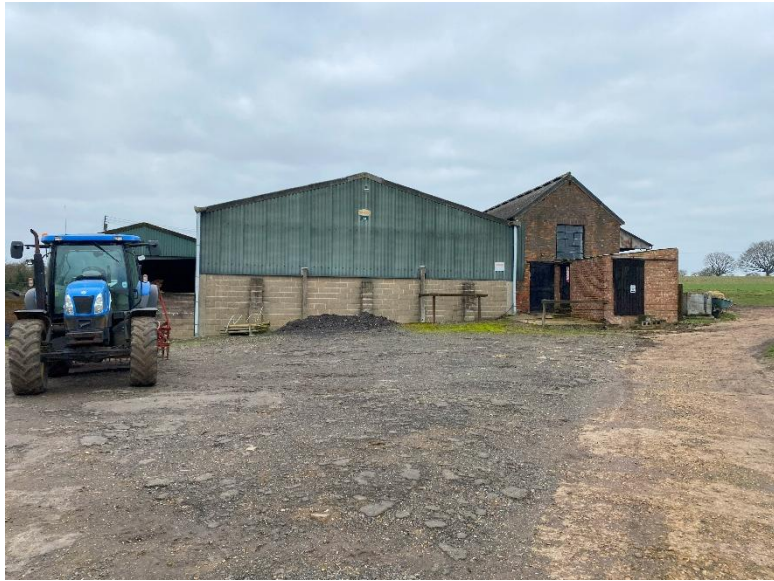
Photograph 1: View looking northwest showing existing agricultural buildings (with green profiled metal and blockwork elevations) for proposed change of use.
