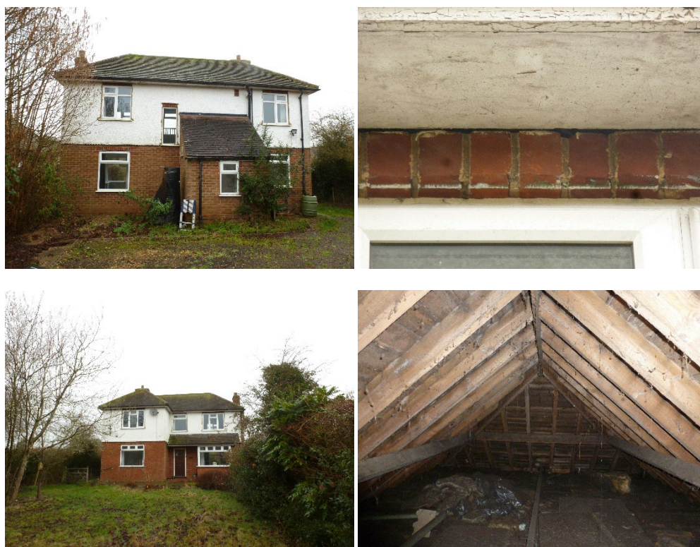
Plates 8 - 11: Photographs of the exterior and interior of the main house, including one of the PRFs identified above the window lintel
