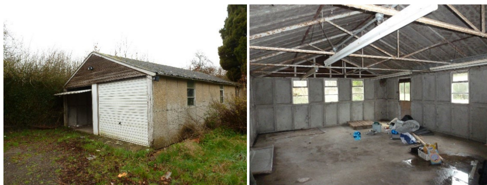
Plates 6 & 7: Photographs of the exterior & interior of the detached garage
