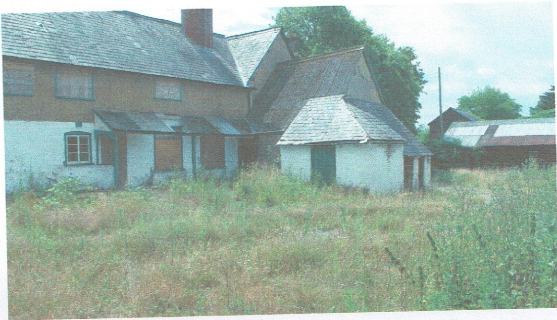
PHOTO No.4 Rear of house with sloping asbestos roof.
