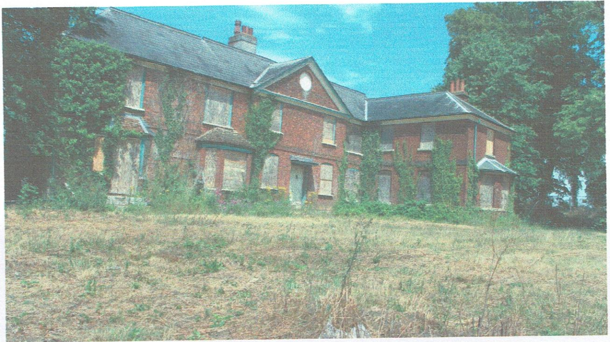
PHOTO No. 15 Building B9 front elevation
