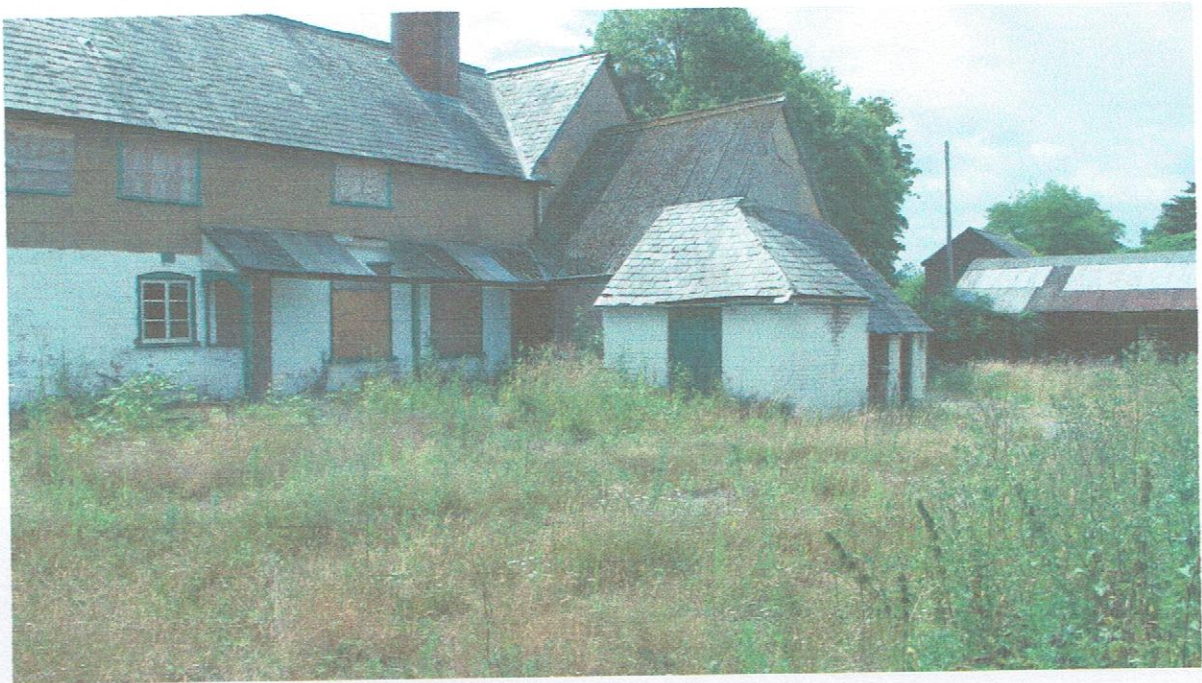
PHOTO No. 16 Building B9 rear with small out building with toilet and kitchen assumed access to basement no further access.
