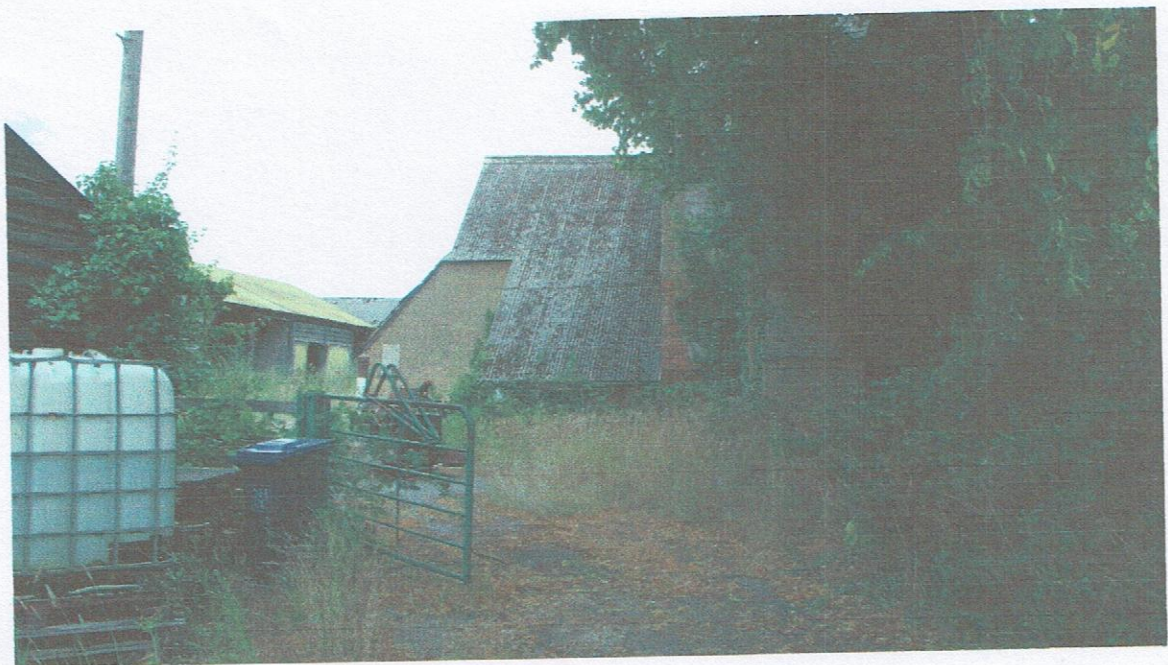
PHOTO No.5 Asbestos roof looking north
