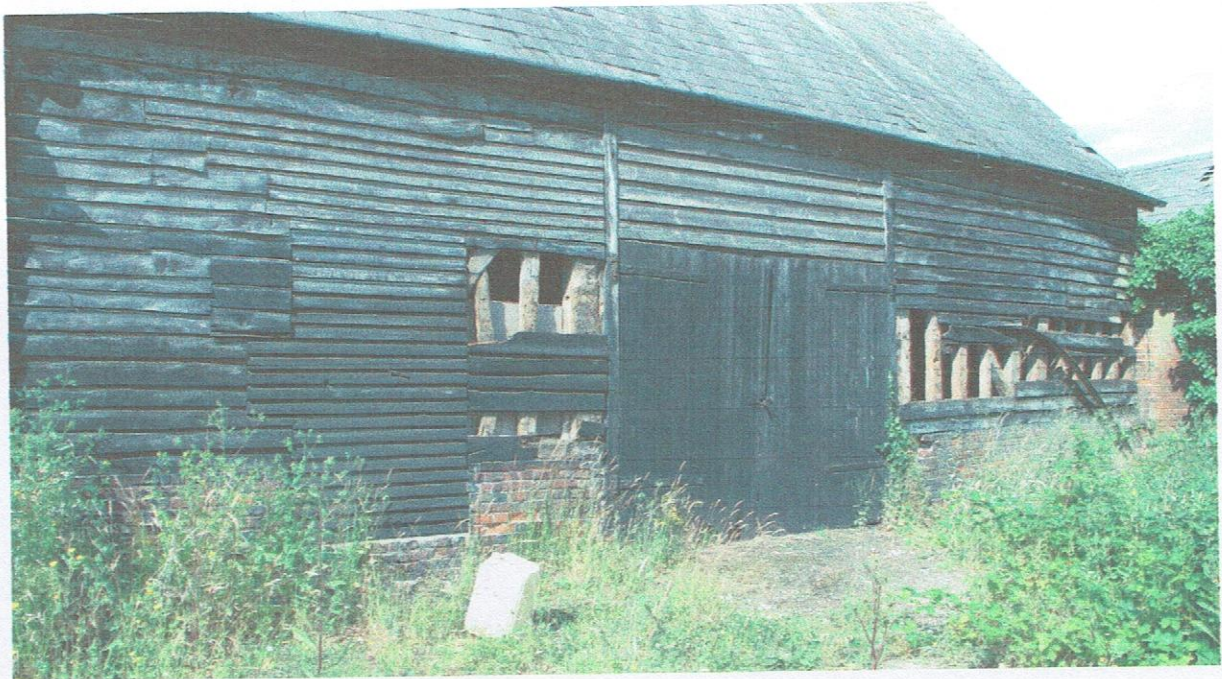
PHOTO No.10 Exterior of Building B4
