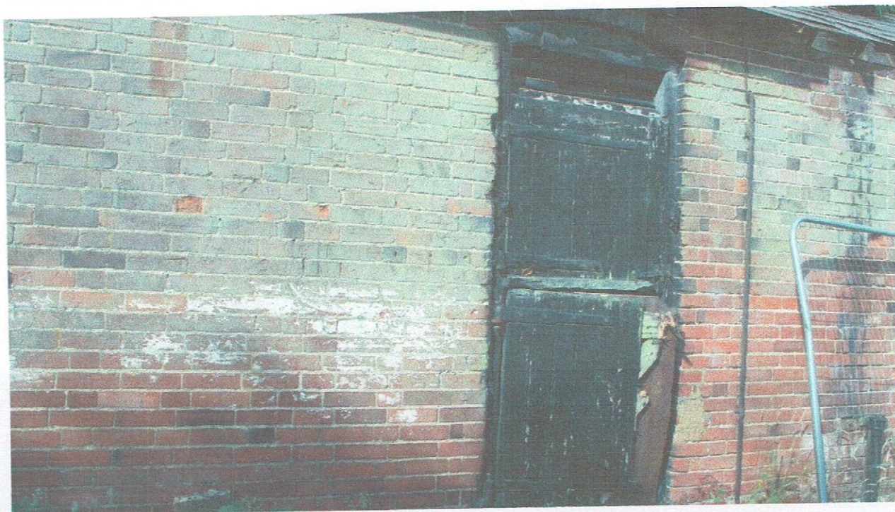
PHOTO No.7 Building B2
