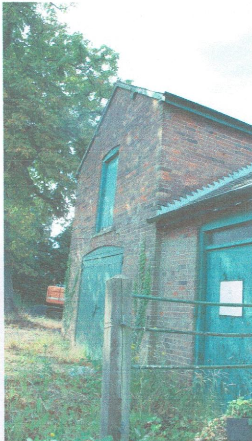
PHOTO No.6 Building B1
