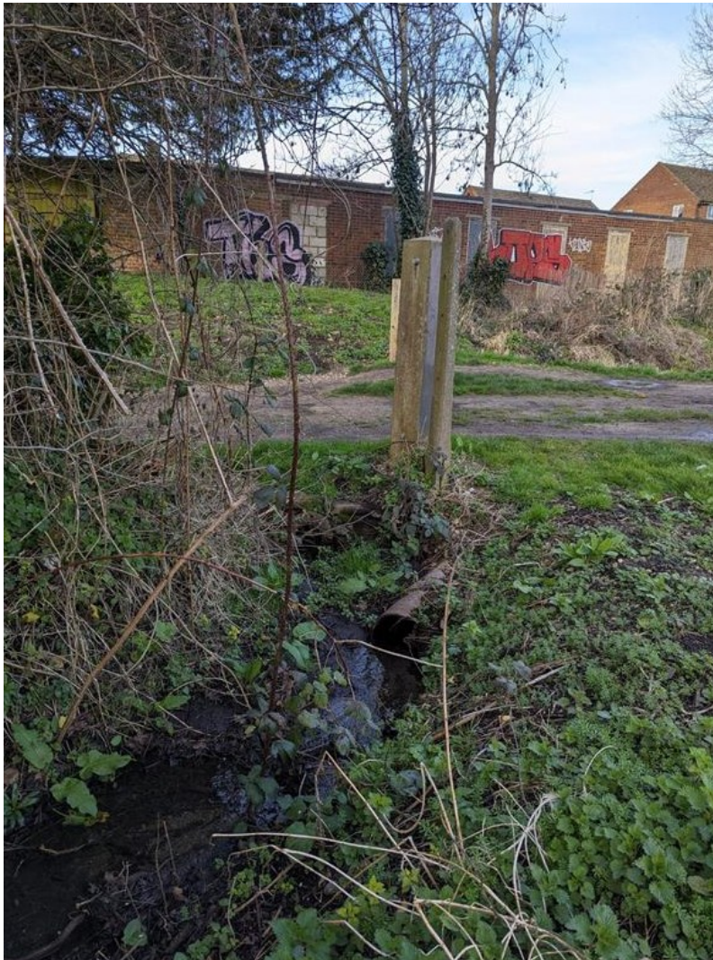
Photo D: Photo looking north at culvert of ditch
