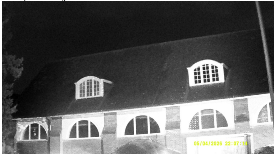
Surveyor IR image: Side elevation - Finish
