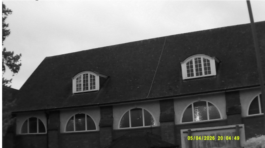
Surveyor IR image: Side elevation - Start
