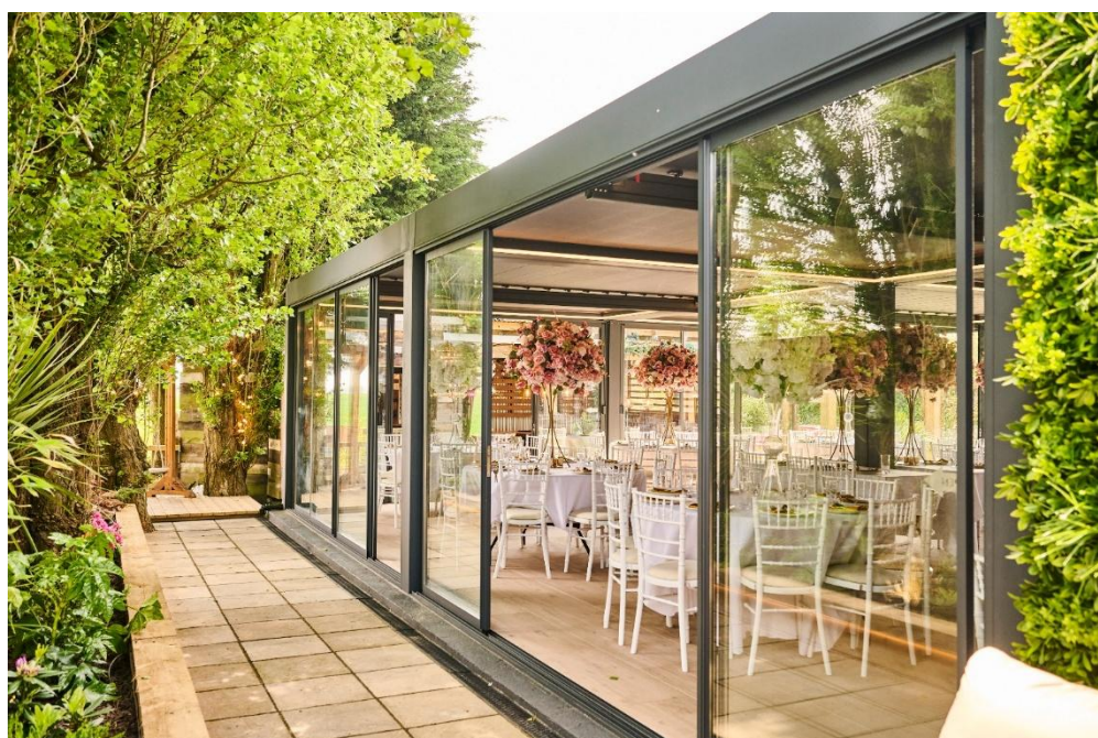
The outside of the new pergola
