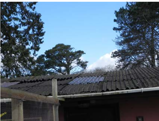
Photograph 9: onduline sloping roof
