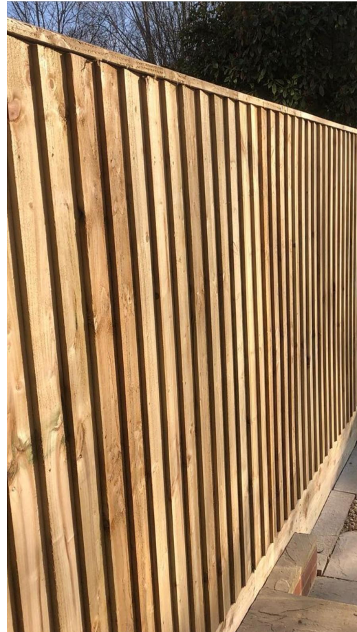
Fence: 1800mm high feather edged timber closeboard fence
