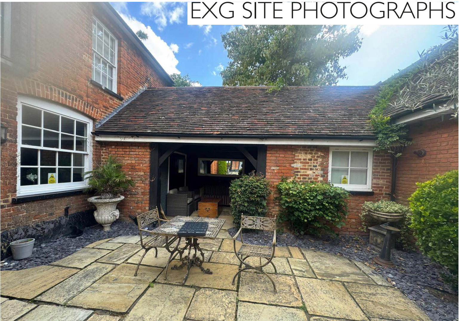
Outhouse/Loggia With Main House Kitchen Window To The Left
