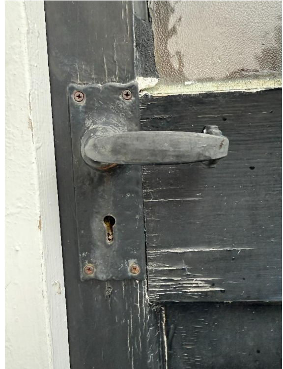
Figure 6 - Internal overview of decay to base of door. Figure 7 - Closeup of mass-produced door handle and obscured glazing/ putty.
