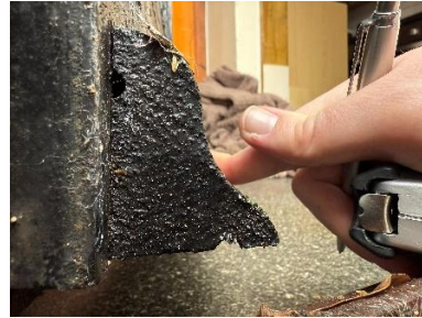
Figure 3 - Profile of existing weathering bar to be retained.
