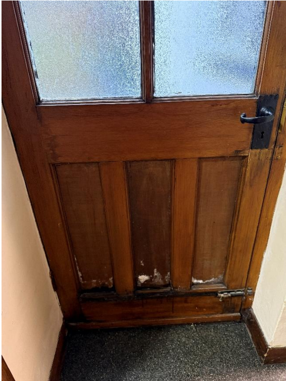
Figure 6 - Internal overview of decay to base of door. Figure 7 - Closeup of mass-produced door handle and obscured glazing/ putty.
