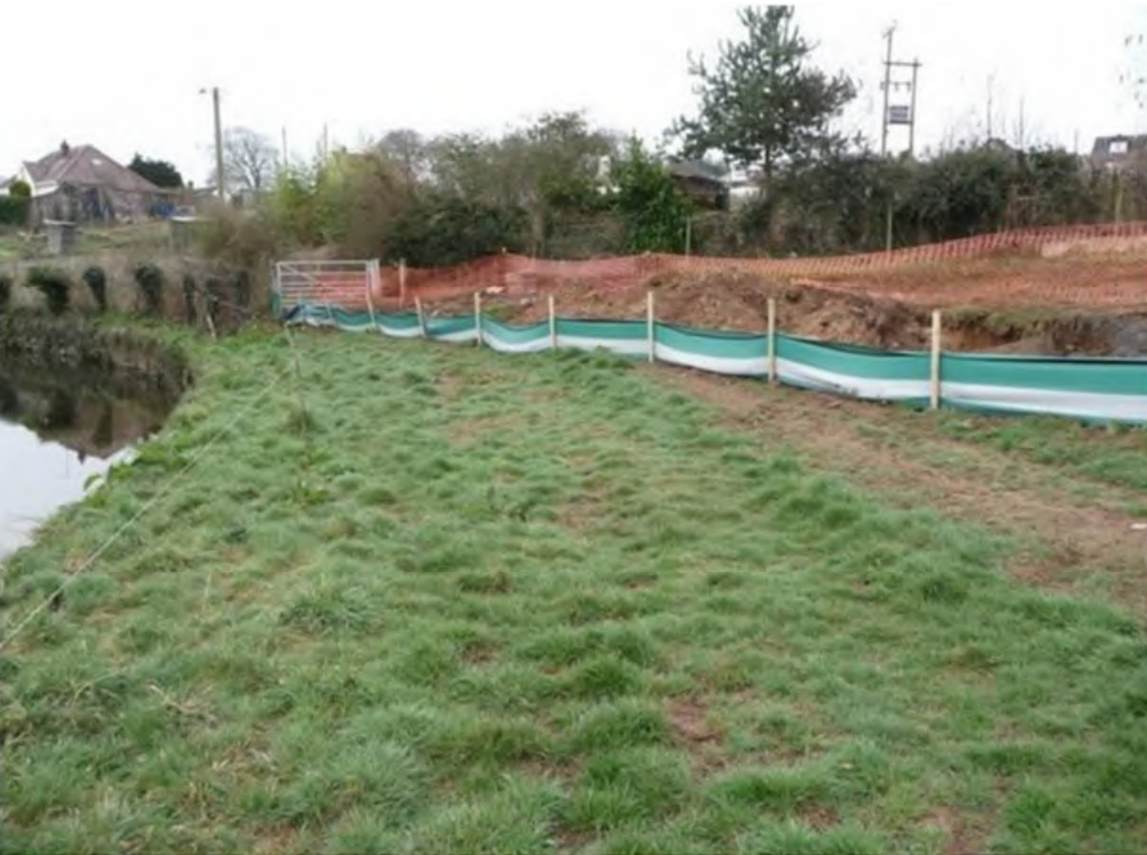
Example of installation of silt fencing and retention of a vegetated buffer zone
