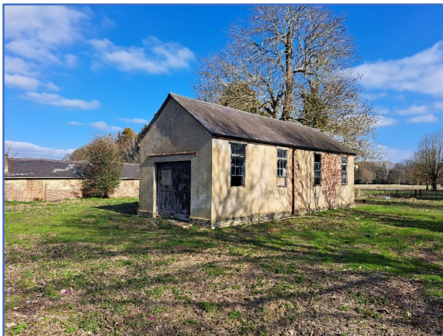
Figure 2 – View of The Old Generator House
