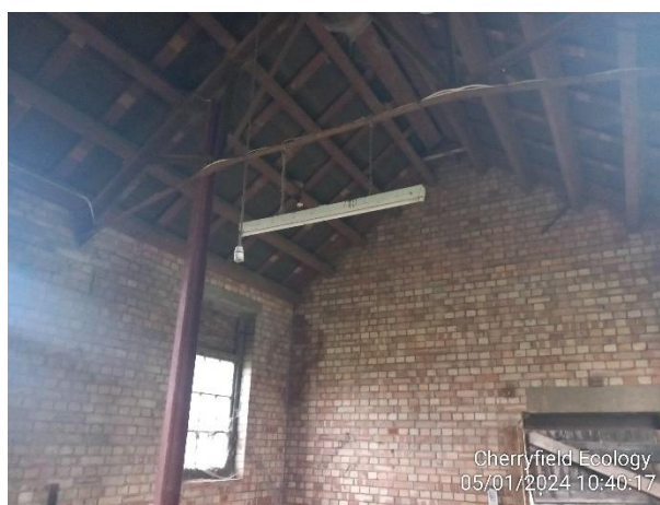
Figure 3: Interior of B1
