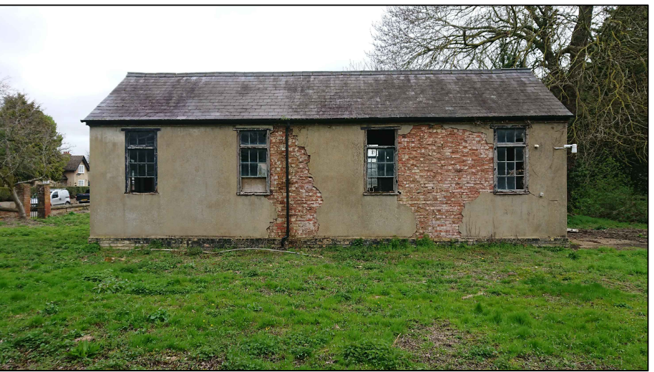
Existing Generator Building Image (South)
