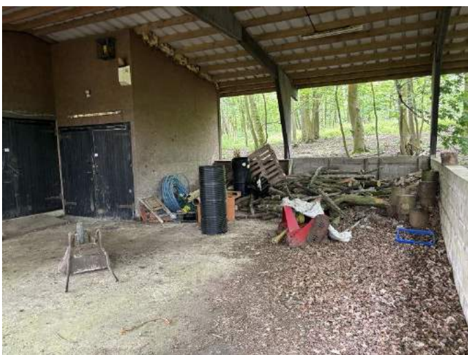
Figure 6: View of the open patio area and stored wood and groundskeeping equipment facing north-east.
