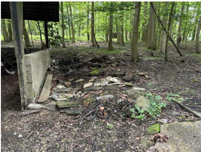
Figure 5: Made Ground to the south of the on-site building facing east.
