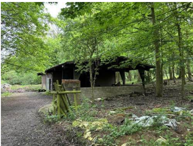
Figure 3: View of the on-site building facing north-east.
