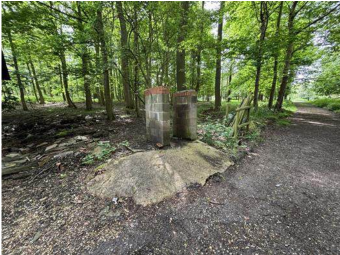
Figure 4: View of the brick and concrete structure facing south-east.
