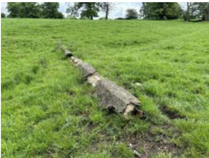
Figure 9: View of the disused drainage features in the north-western section of the site facing north-west.
