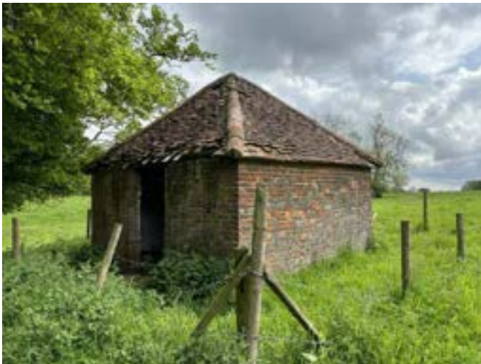
Figure 8: View of the piggery facing north.
