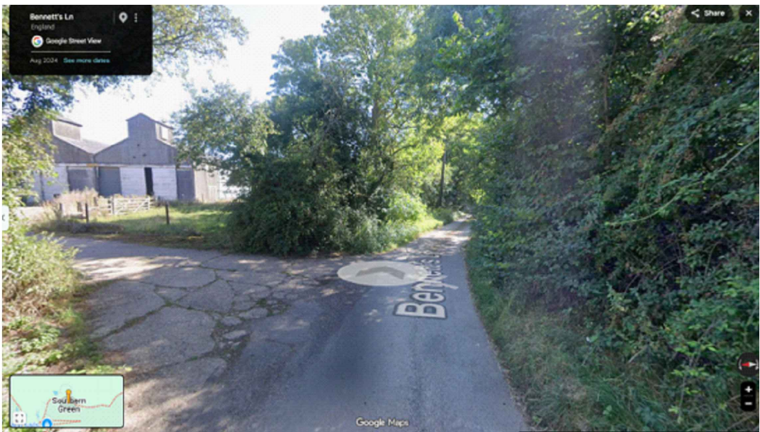
Street view looking East
