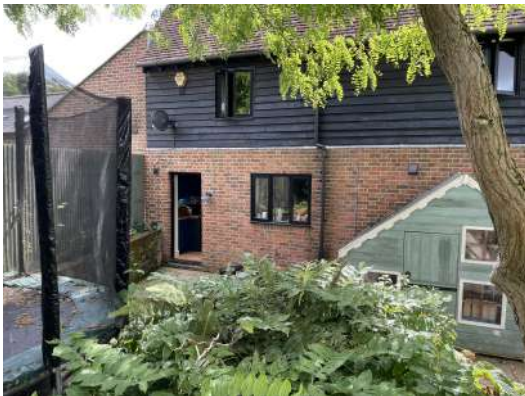
Rear elevation of Daubentons Barn showing the non-historic cavity masonry wall up to first floor level.
