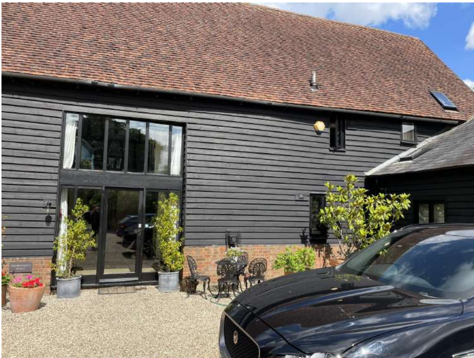
Daubentons Barn – west (front elevation)
