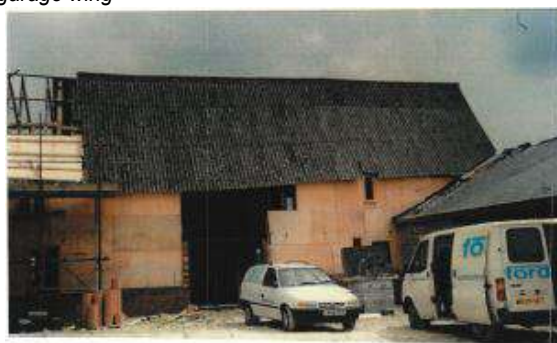
Daubentons Barn with the timber frame bracing being added and openings appearing.
