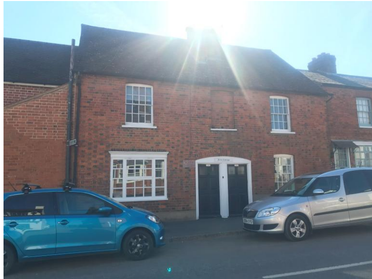
Figure 9 – 126 and Fern Cottage
