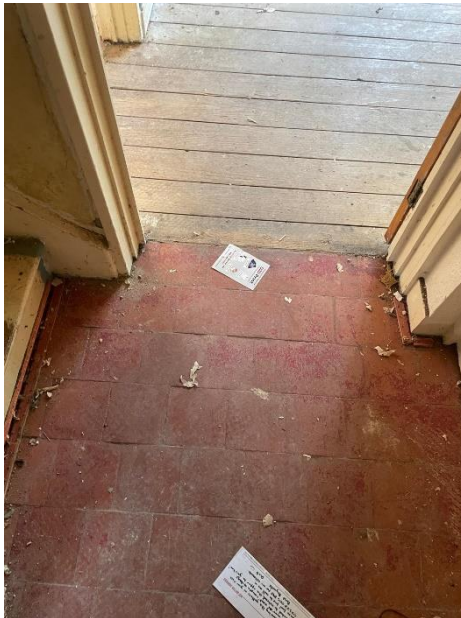
Picture 5 – Juxtapose of differing floor finishes and construction.
