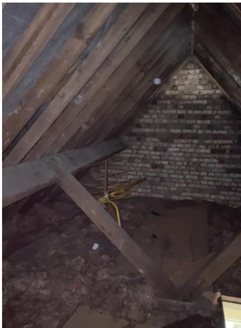
Picture 6 and 7 – Unventilated roof void, and extensive lowered eaves sections.
